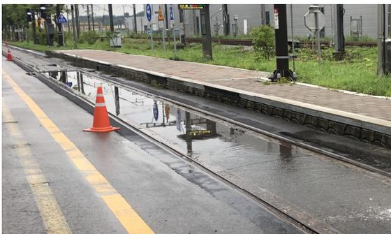
**Fig. 14.** water-reservoir phenomenon in rainy situation
