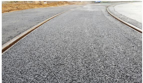
**Fig. 13.** Surface of asphalt pavement of embedded track system
