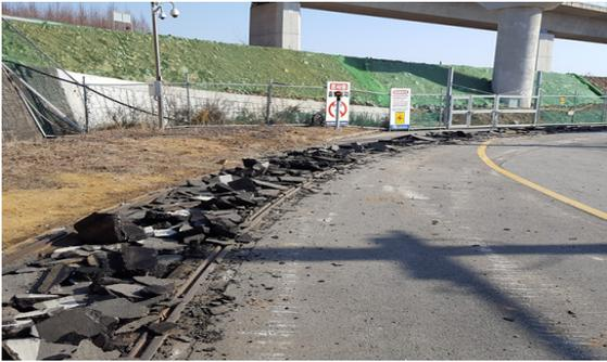
**Fig. 10.** Crushing of existing asphalt concrete
