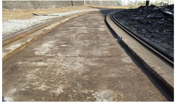
**Fig. 11.** Cleaning of embedded track system for tram
