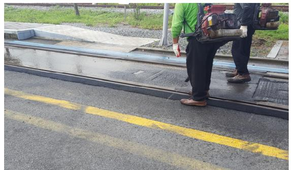
**Fig. 15.** moisture removal on site
