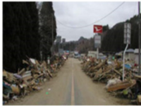
Road opening through restoration
