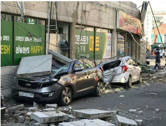
(a) destruction of build wall
